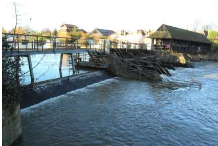
Plate 2-11: Photograph of the existing overfall weir (far left) on weir C at Molesey.
