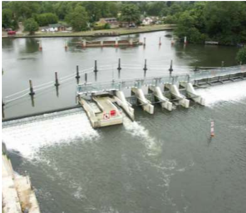
Plate 2-6: An example of a typical flow control structure.
