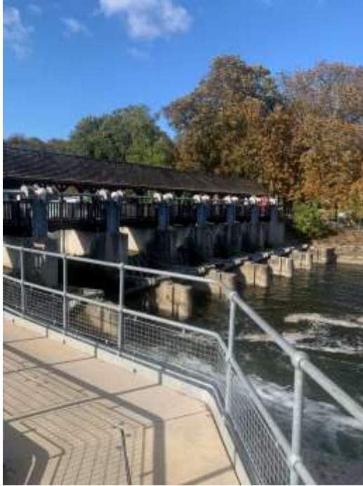
Plate 2-10: An example of an existing River Thames radial gate weir at Molesey.
