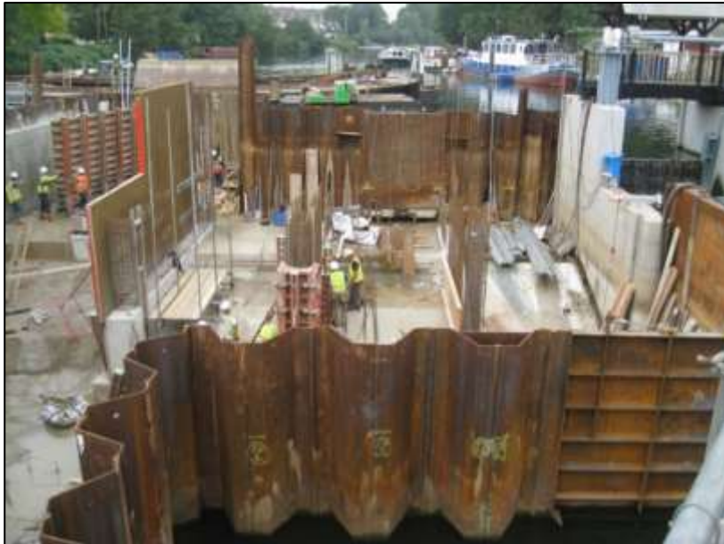
Plate 2-17: An example of a cofferdam, used to construct new weir gates.
