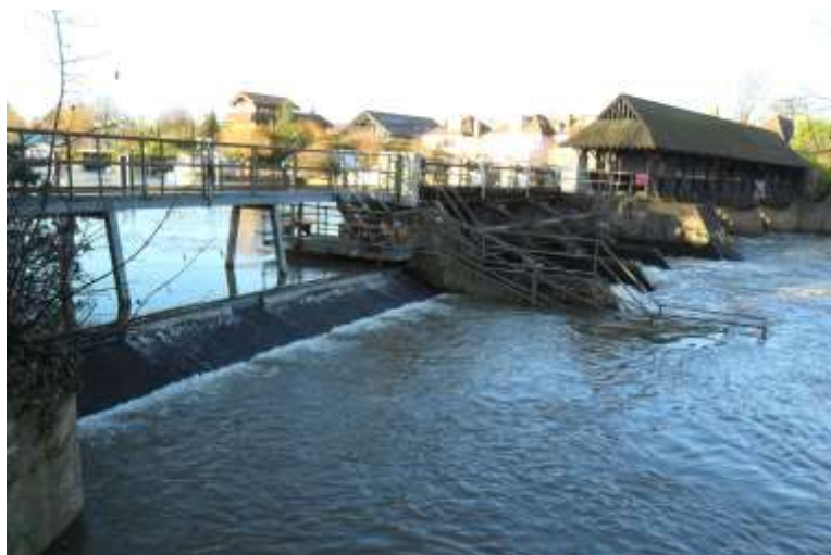
Plate 2-11: Photograph of the existing overfall weir (far left) on weir C at Molesey.
