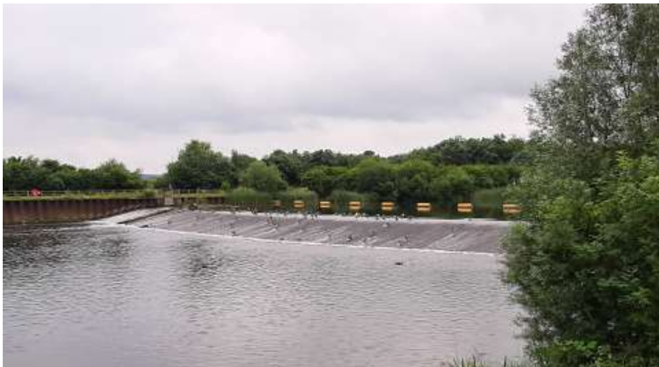
Plate 2-7: An example of a typical water level control structure.
