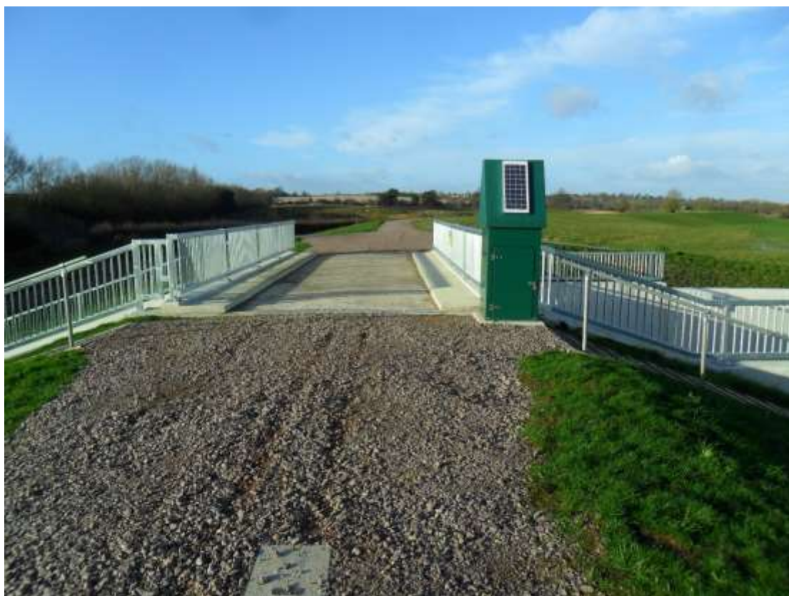
Plate 2-16: An example of an accommodation bridge
