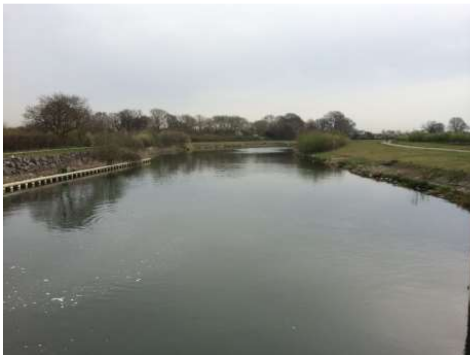
Plate 2-1: An image of the Jubilee River, which provides an impression of how the flood channel will look
