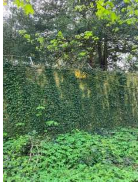
Plate 10. Pond 33 has a 3m high wall around pond. Unable to conduct HSI assessment.
