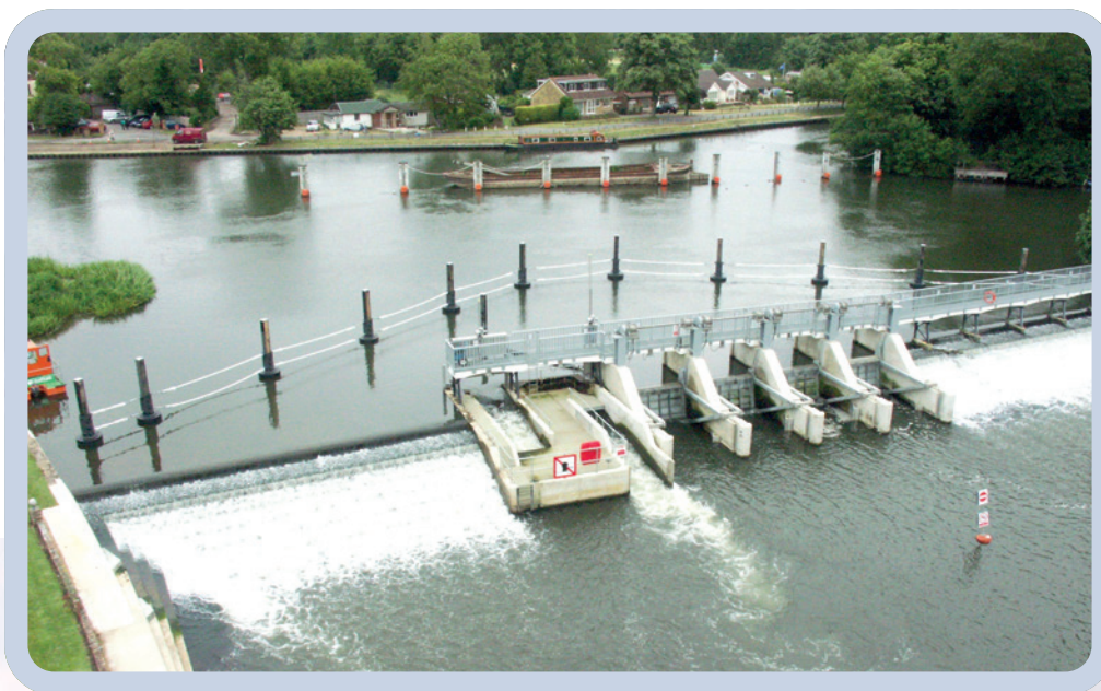
Above: Shep Weir Below: Manor Farm Weir
