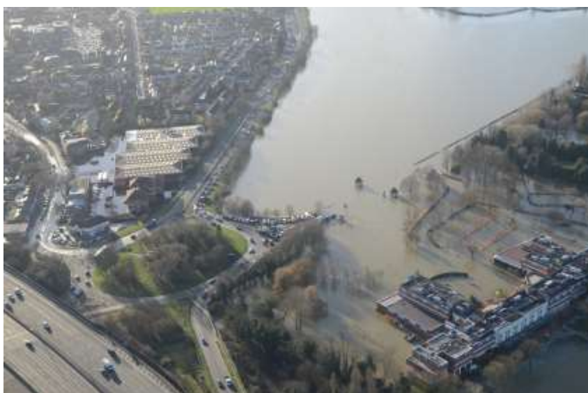
Plate 1: Flooding at Runnymede (M25 junction 13) in 2014
