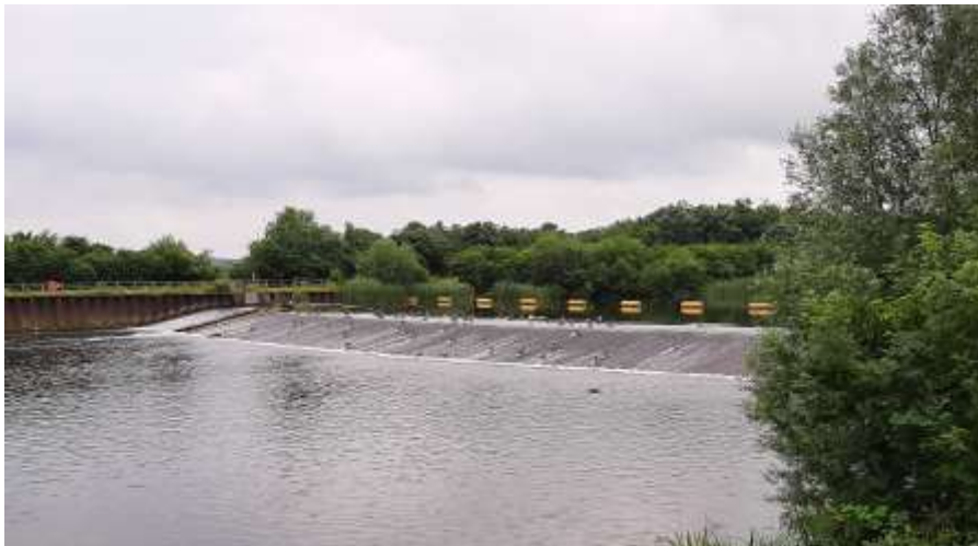
Plate 4: An example of a water level control structure
