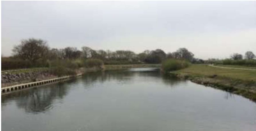
Plate 3: An image of the Jubilee River, which provides an impression of how the RTS flood channel will look
